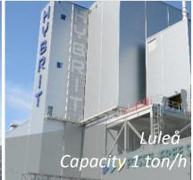
H<sub>2</sub> replacing C for iron ore reduction, resulting in H<sub>2</sub>O instead of CO<sub>2</sub>
